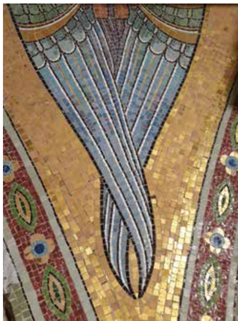
Fig. 1. Altered, randomly located gold leaf tesserae in situ . of mosaics in the dome and the pendentives by Zsigmond Vajda and Miksa Róth. In 1904. South-Eastern dome of the Archways by Lajos Gerle in the Fiumei Road National Cemetery, Budapest (photo by B. M. Kürtösi)
