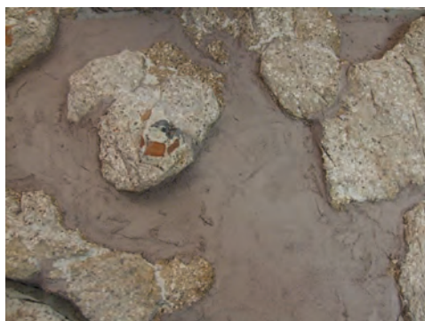
Fig. 11. The leveling of the backside of the mosaic was made by the lightweight lime-based mortar (Photo: Brigitta Maria Kürtösi)
